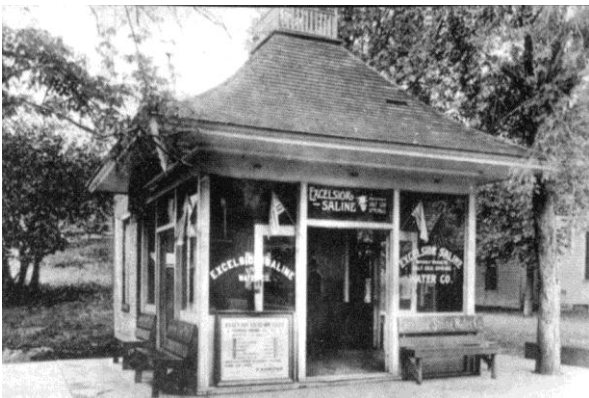
Historic photo of Excelsior Saline pavilion with masonry addition at rear
