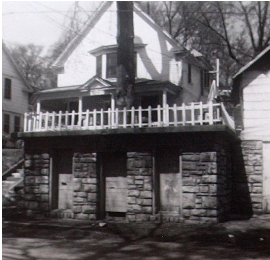
Historic photograph of sales pavilion on Caldwell
